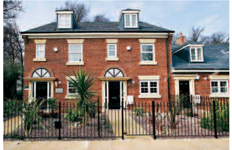
Farington Villas, Farington, Lancashire
